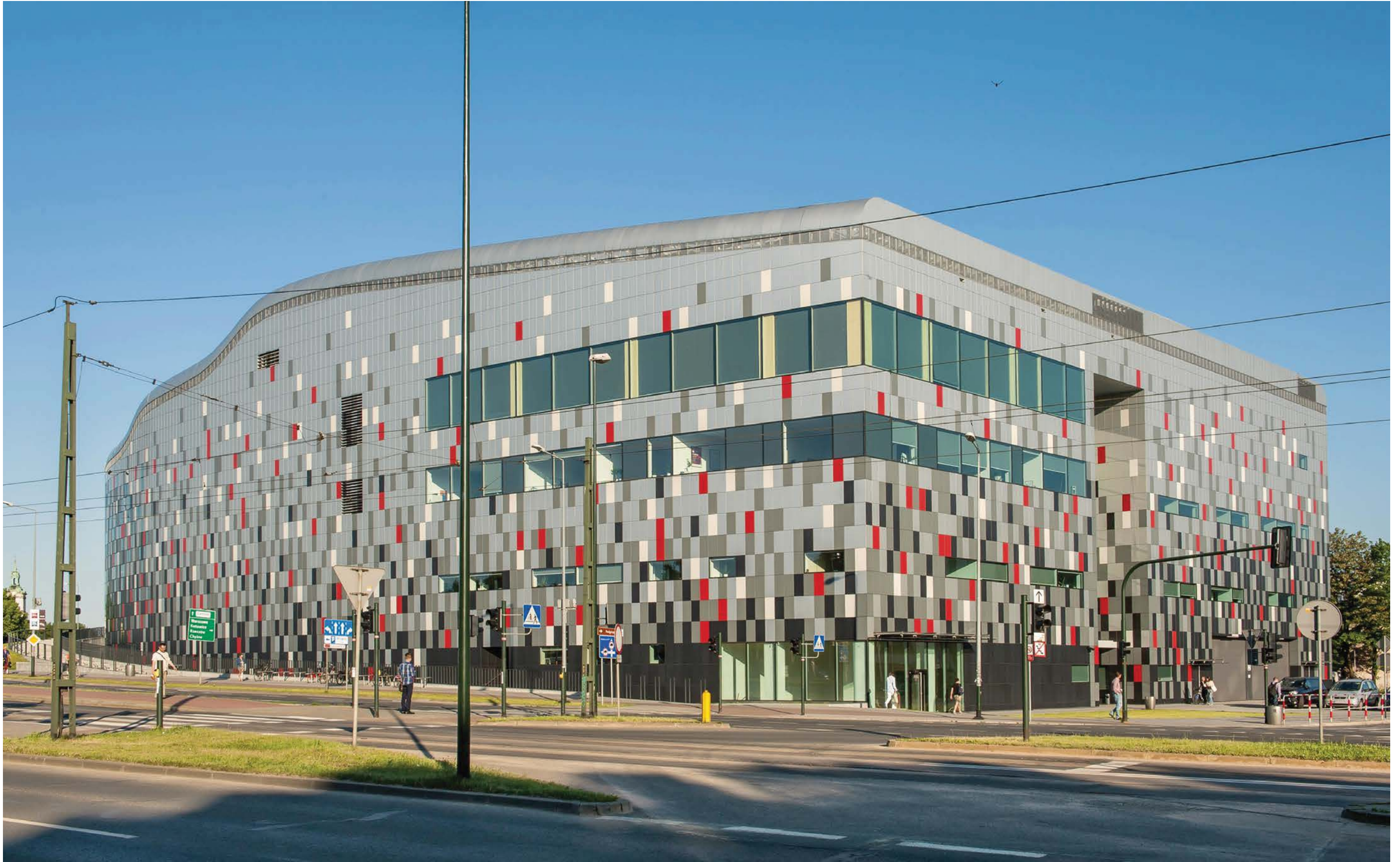
ICE Cracow Congress Center, Cracovia, Poland. Project: Ingarden & Ewa Architekci SistemA Nero, Rosso, Grigio
