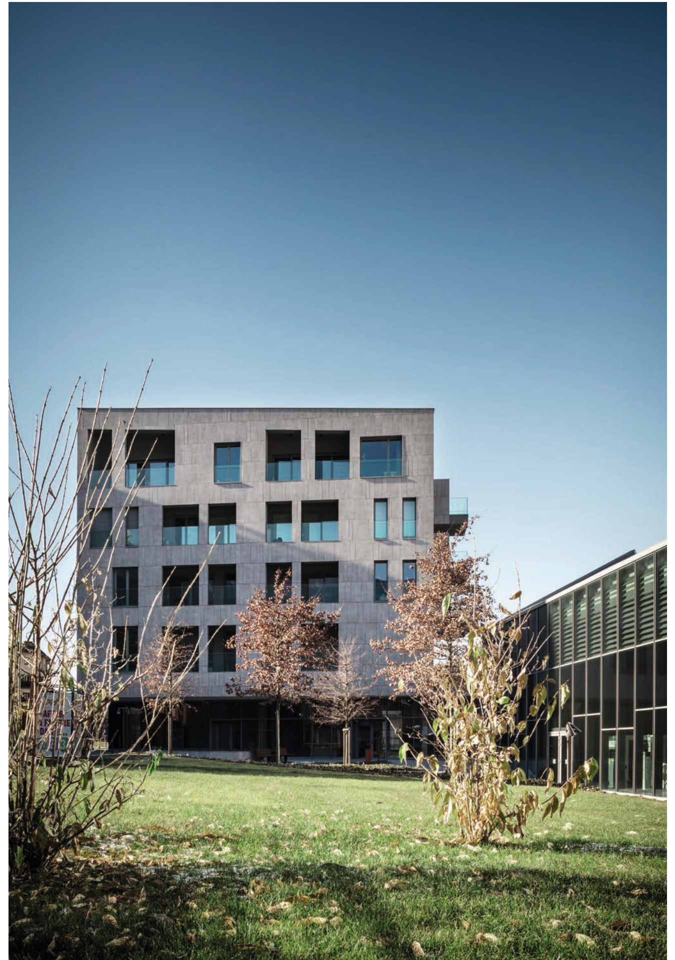
Ex Martinelli Building, Morbegno (SO) Italy. Project: Antonio Citterio Patricia Viel
