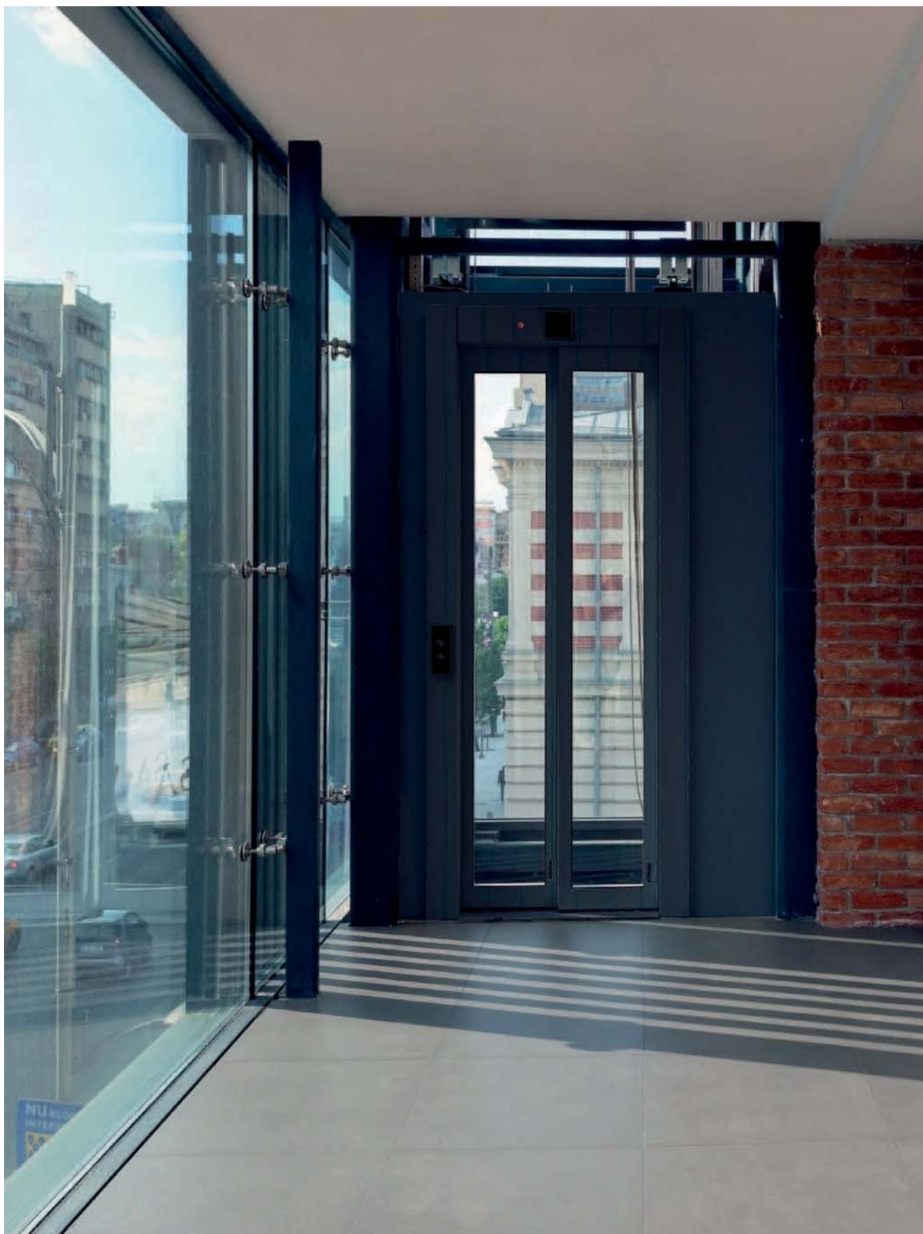
Media One Building, Bucharest, Romania. Project: Cristina Georgescu M826 SistemN Grigio Medio 60x60
